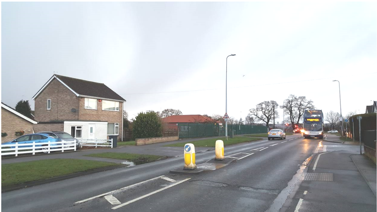
View northeast along Birchwood Avenue and the site frontage
